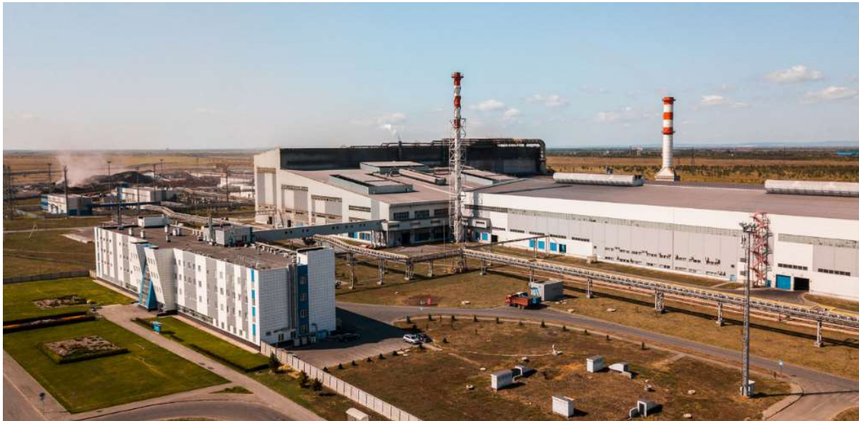
AO Steel Works Balakovo in Saratov region, Russian Federation
