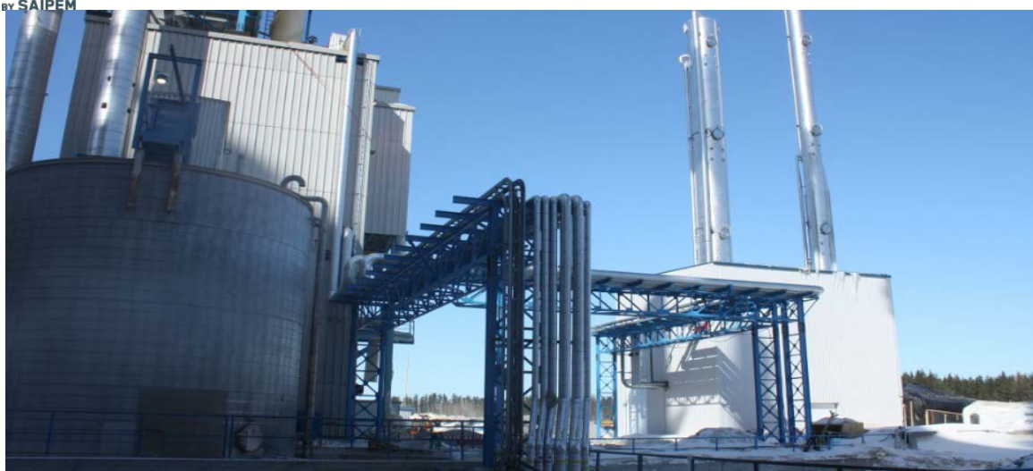
CO 2 Capture Plant of 30 tons per day operating on a commercial scale at Saint-Felicien, Quebec, Canada
