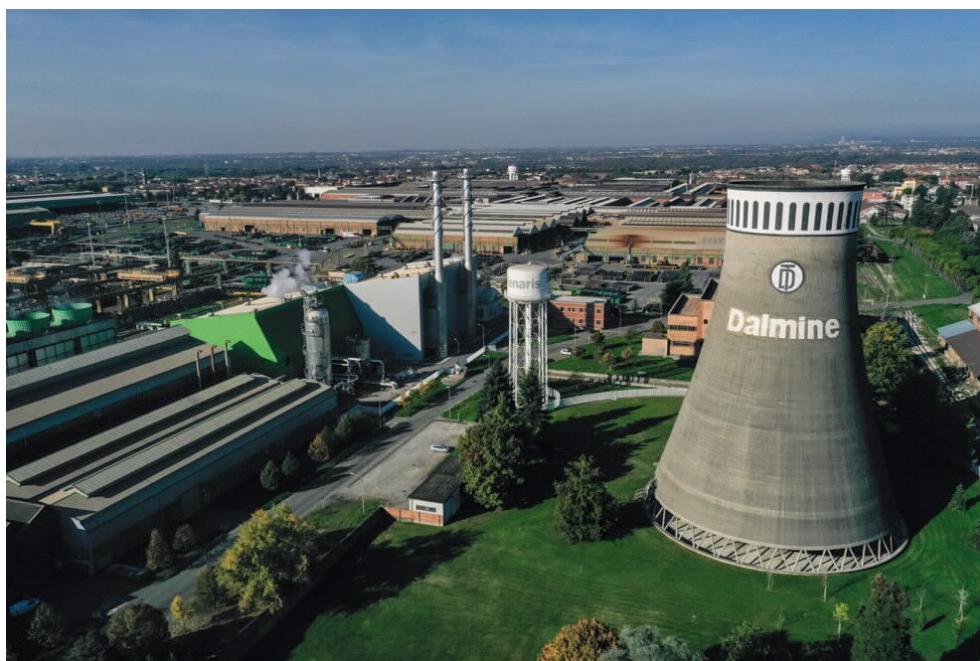
Area of the TenarisDalmine plant where (on the left) the thermoelectric plant is located
