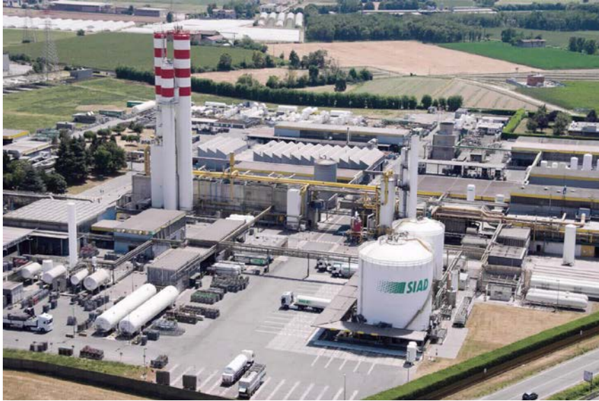
The Osio Sopra (Italy) plant, the main SIAD production center, is the largest and most comprehensive national facility in the industrial gas sector
