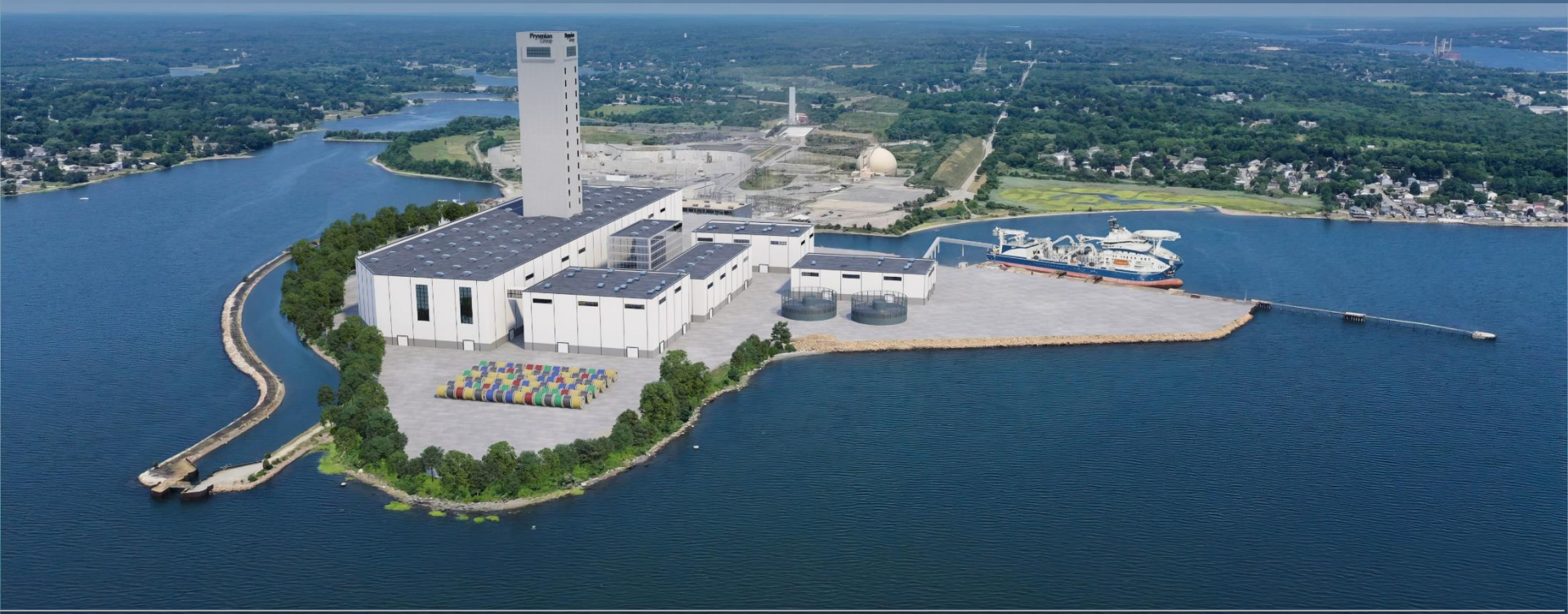
New submarine cable plant in Brayton Point, Massachusetts, USA
