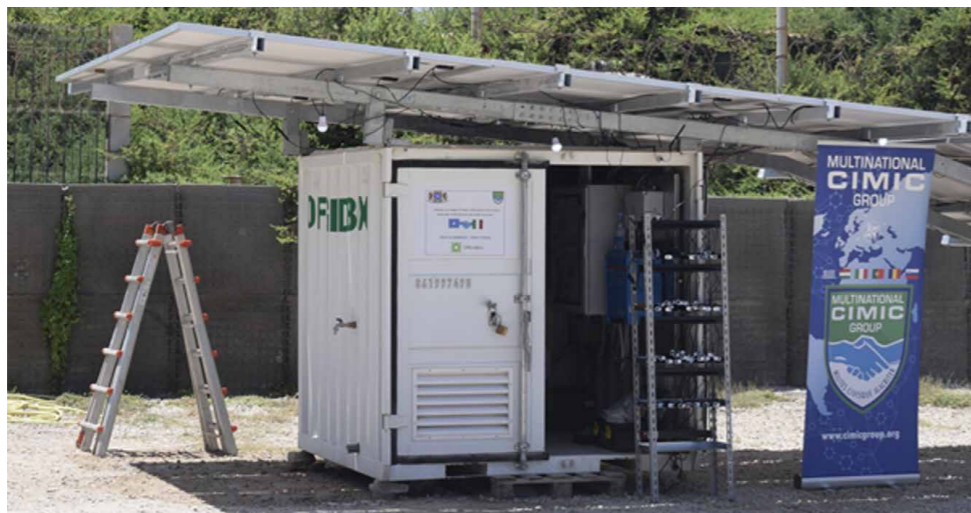
Figure 22: A box from La Fabbrica del Sole with SECO solutions installed in Somalia
