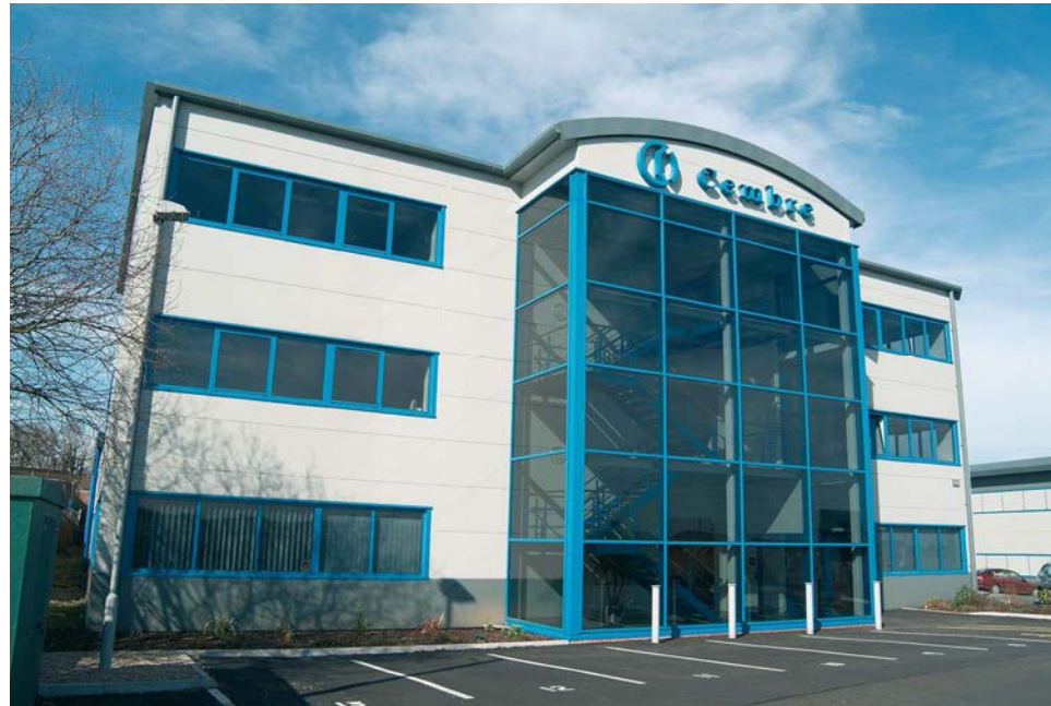
Cembre Ltd. Factory in Curdworth Birmingham (UK)
