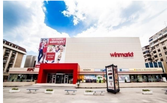
Ploiesti Omnia: facade restyling nearly completed
