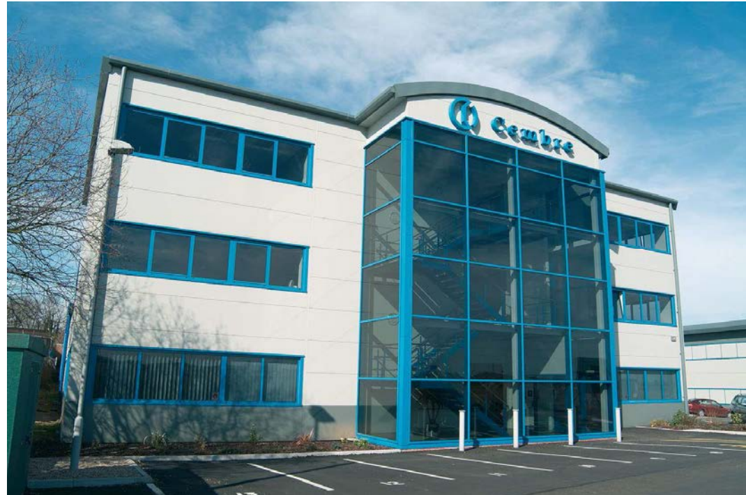
Cembre Ltd. Factory in Curdworth Birmingham (UK)
