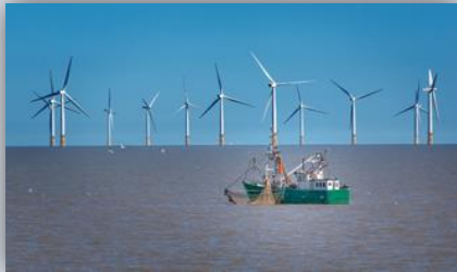
Offshore wind farm
