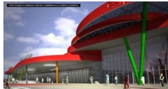
ESP – Ravenna Extension 1H 2017 ~ €53 mn total
