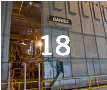
Dog-house and Elephant-house structures for EAF noise control
