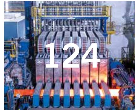
QHeat induction heating & converters
