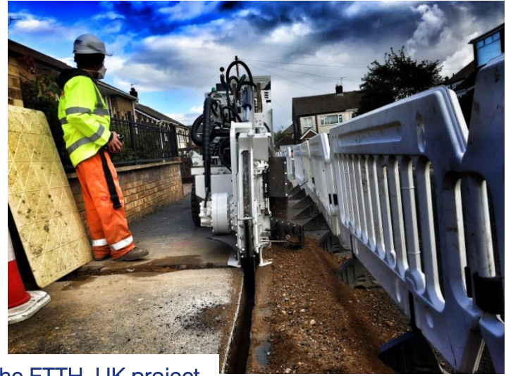
Side cut working on the FTTH UK project
