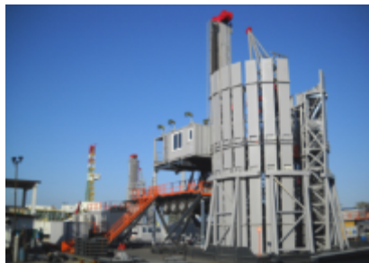
Hydraulic Drilling Rigs
