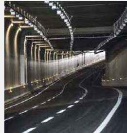
Tunnels and underground works
