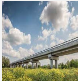
Road and Railway infrastructures
