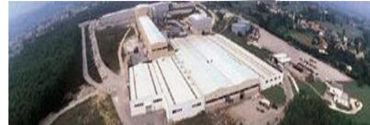
Santa Giustina's plant
