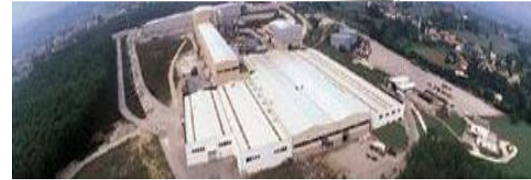
Santa Giustina's plant
