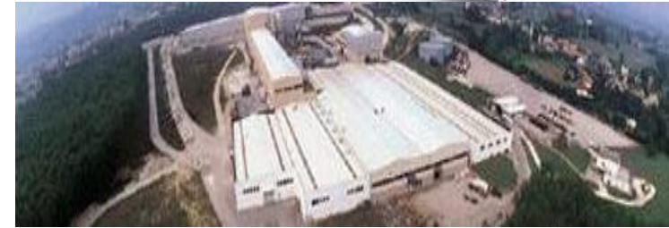
Santa Giustina's plant
