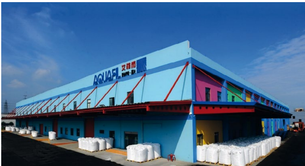
Figure 17 - Visual impact of the Chinese JIAXING plant
