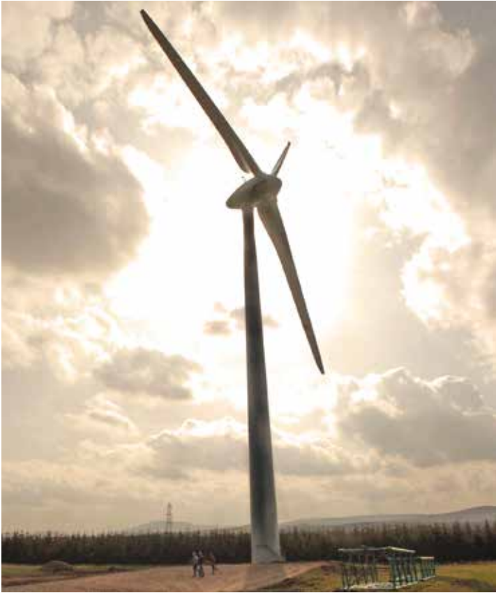
Boyndie (Great Britain) wind farm
