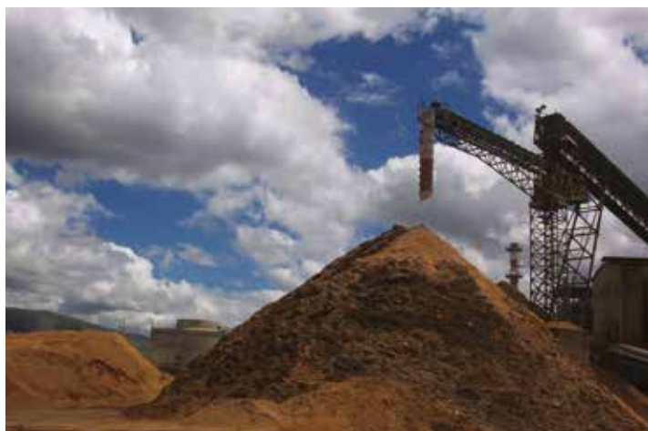
Rende (Cosenza) biomass and photovoltaic plant
