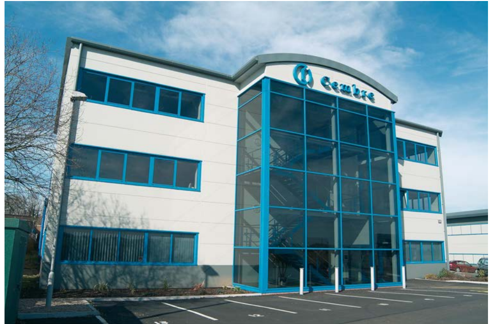
Cembre Ltd. Factory in Curdworth Birmingham (UK)
