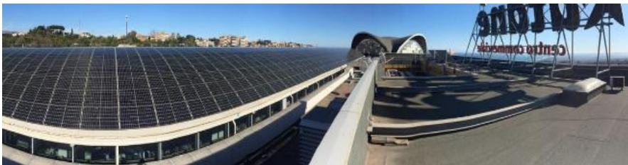
New photovoltaic system in Katanè
