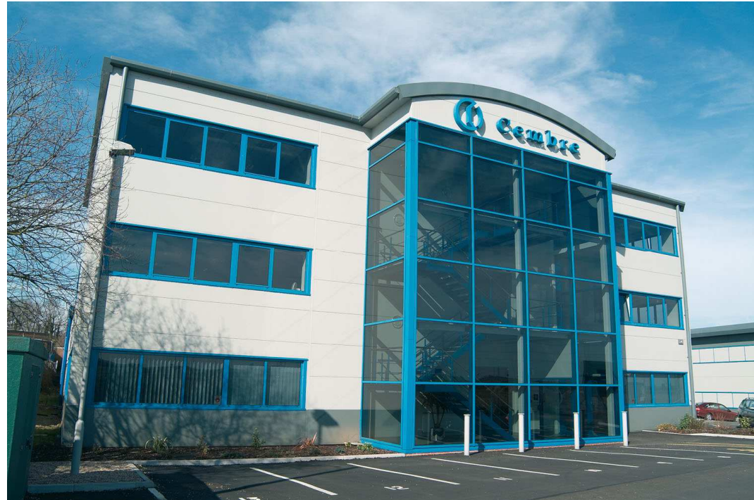
Cembre Ltd. Factory in Curdworth Birmingham (UK)
