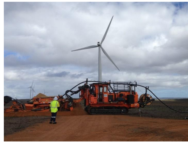
Wind and Solar Farms Automatic cables laying system
