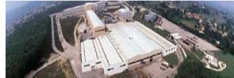
Santa Giustina plant
