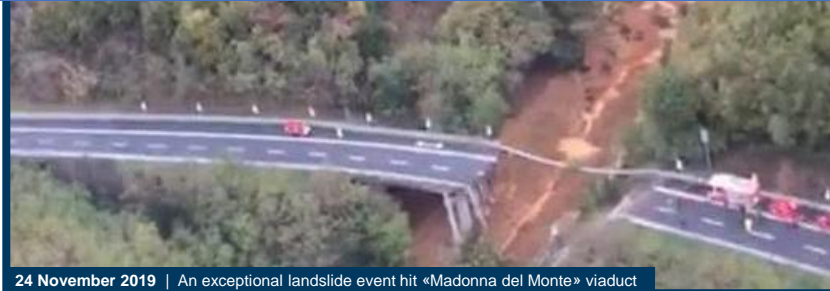
24 November 2019 | An exceptional landslide event hit «Madonna del Monte» viaduct
