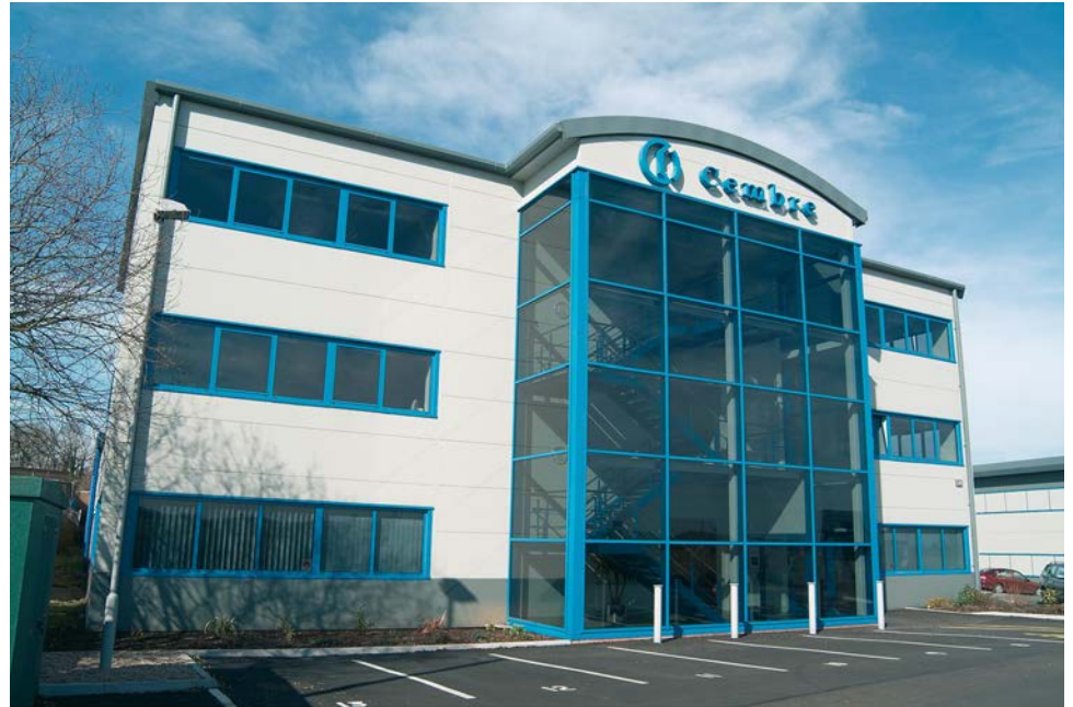
Cembre Ltd. Factory in Curdworth Birmingham (UK)
