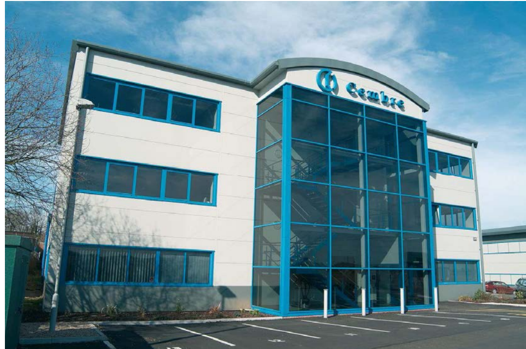
Cembre Ltd. Factory in Curdworth Birmingham (UK)
