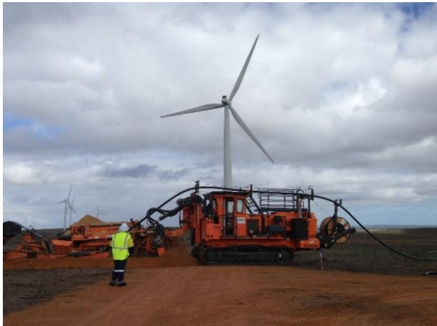
Wind Farm (Australia) Automatic cables laying system
