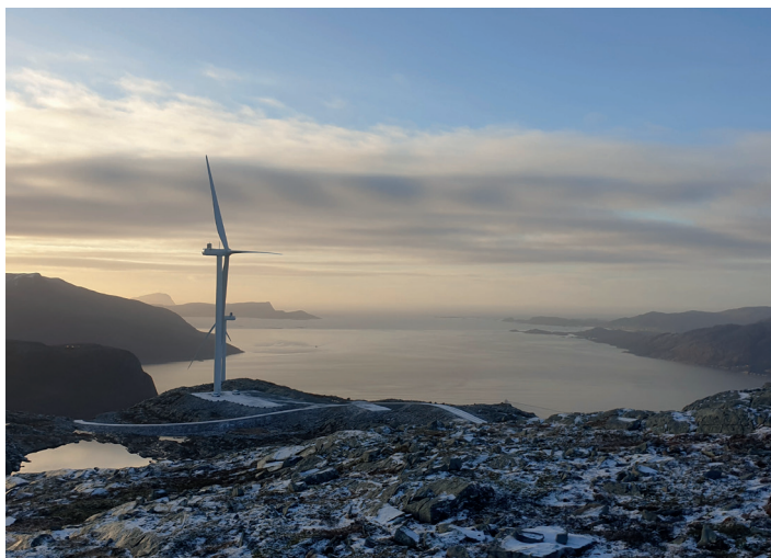
Hennøy (Norway) wind farm
