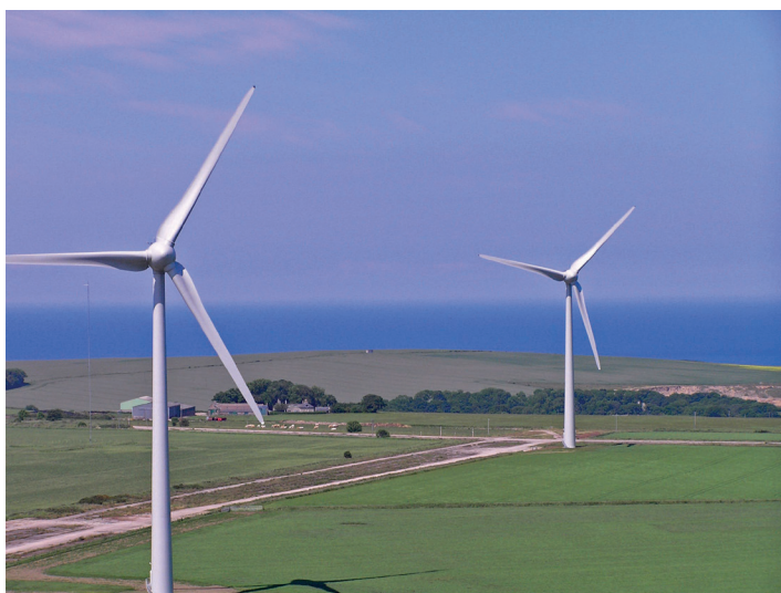
Boyndie (Great Britain) wind farm
