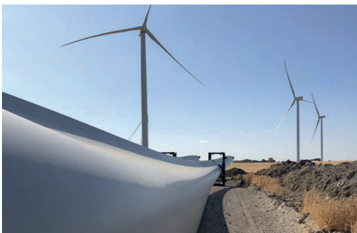
Carreastro (Spain) wind farm
