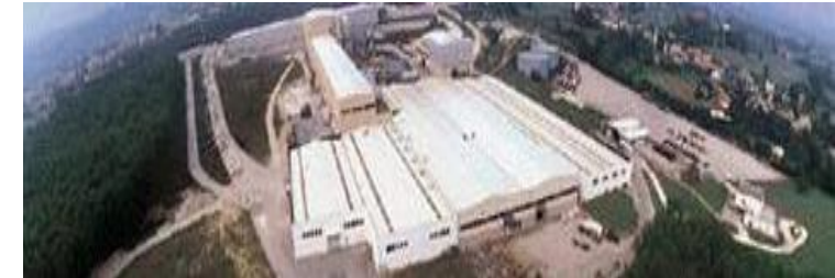
Santa Giustina plant
