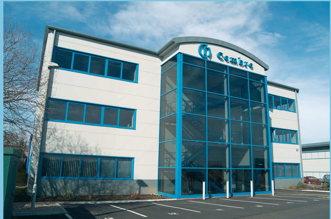
Cembre Ltd. – Factory in Curdworth Birmingham (UK)
