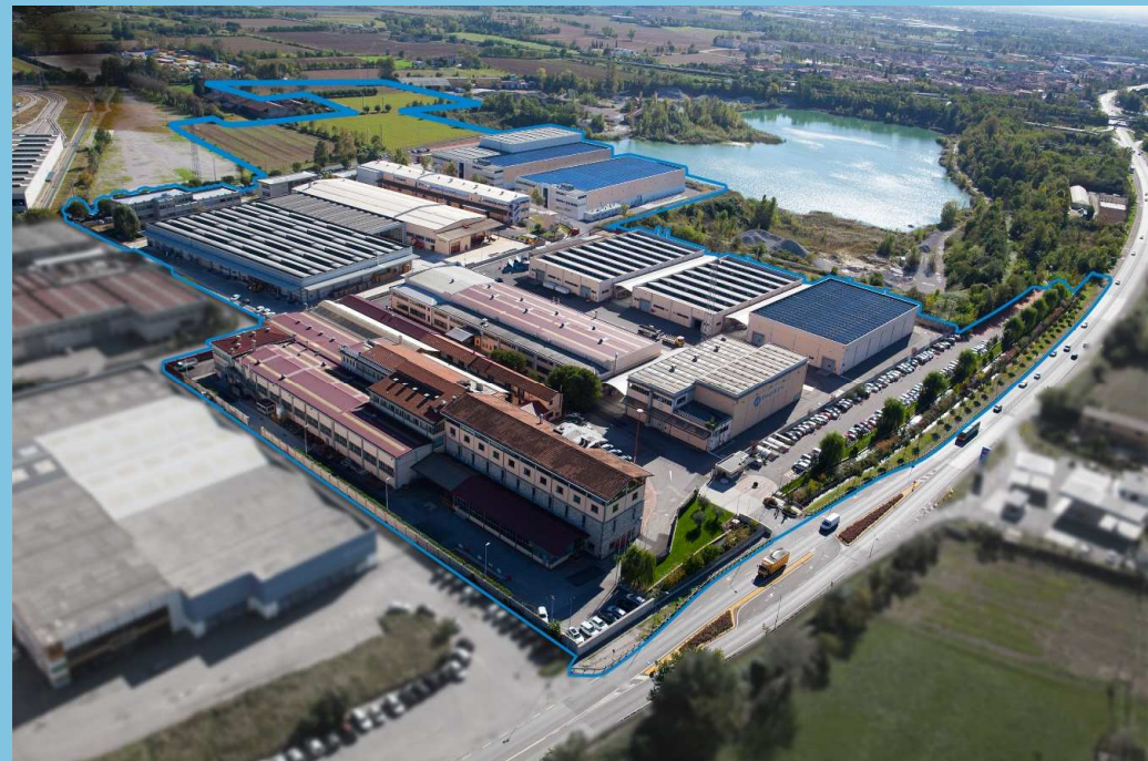
Cembre S.p.A. – Headquarter in Brescia (Italy)
