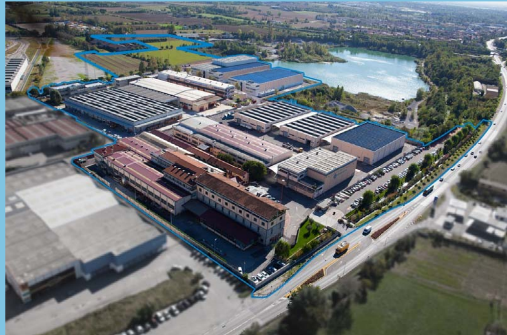
Cembre S.p.A. – Headquarter in Brescia (Italy)
