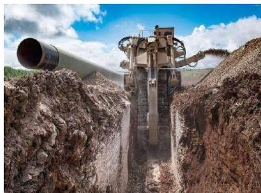
Figura 7 – *Trencher a catena – Chainsaw*
