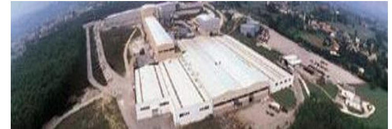
Santa Giustina plant
