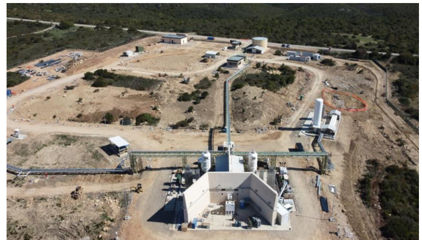
SPTF facility under construction in Sardinia
