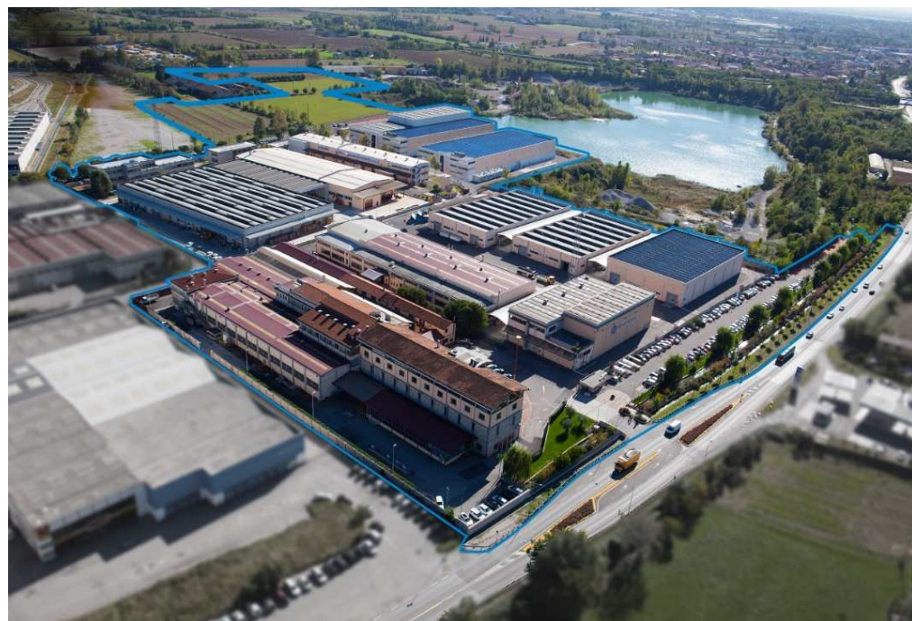
CEMBRE S.p.A. – Headquarter in Brescia (Italy)
