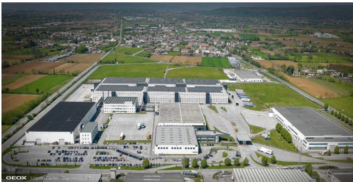
External warehouses and the Signoressa logistics hub
