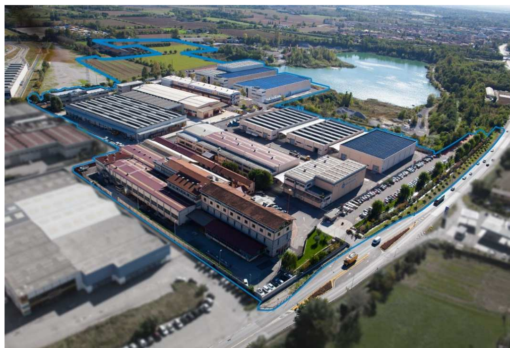
CEMBRE S.p.A. – Headquarter in Brescia (Italy)
