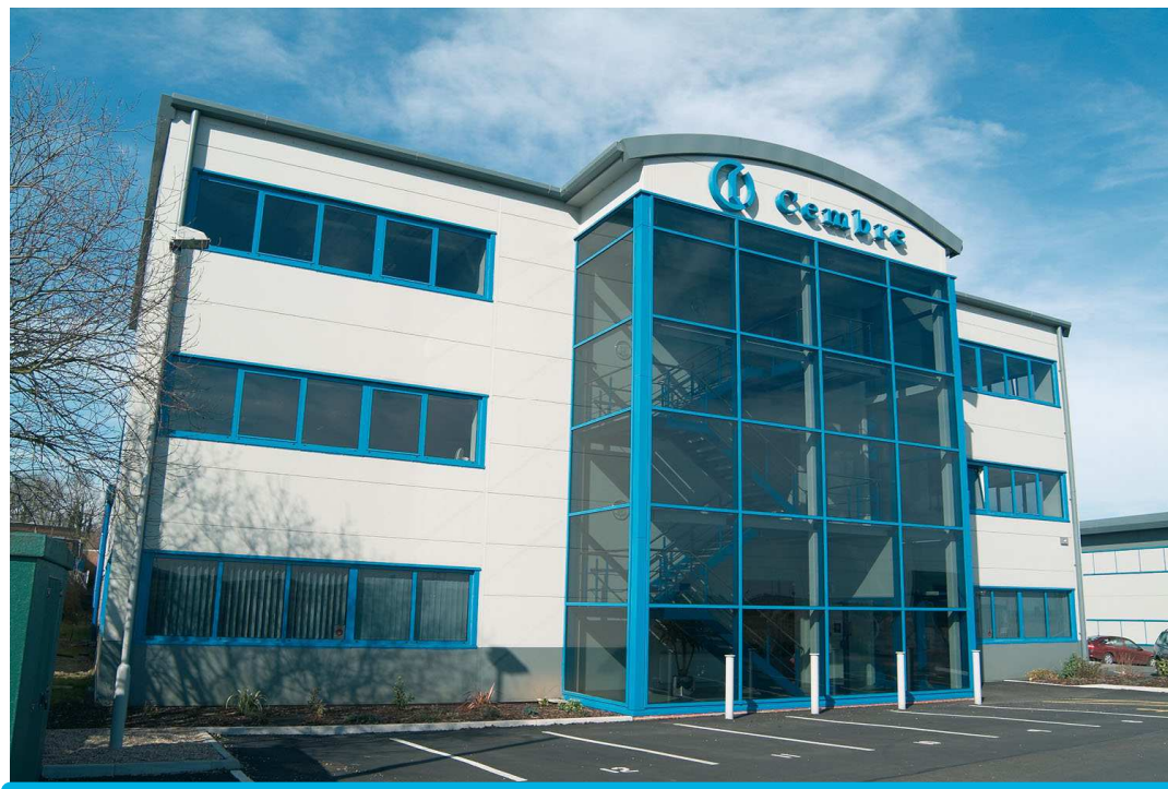
CEMBRE Ltd. – Factory in Curdworth Birmingham (UK)
