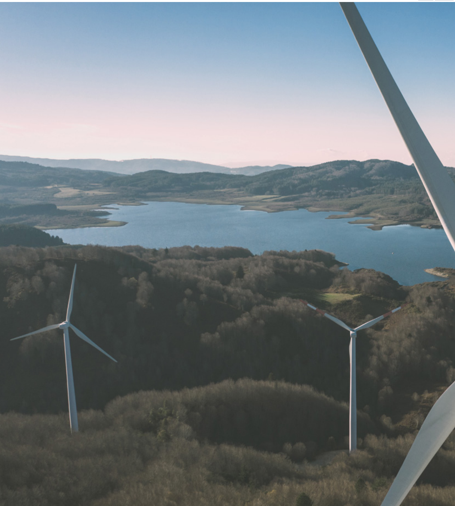
San Sostene (CZ) wind farm.
