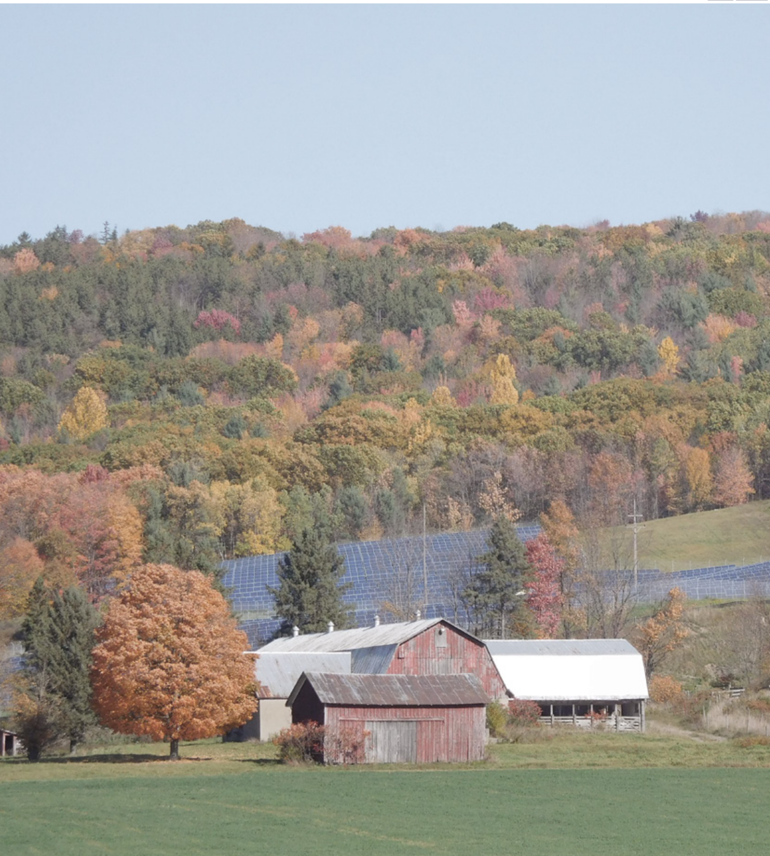
Harford - Davi (USA) photovoltaic plant.
