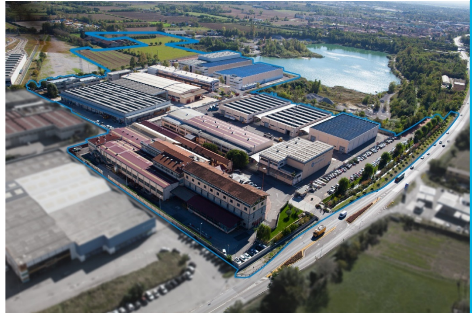
CEMBRE S.p.A. – Headquarter in Brescia (Italy)
