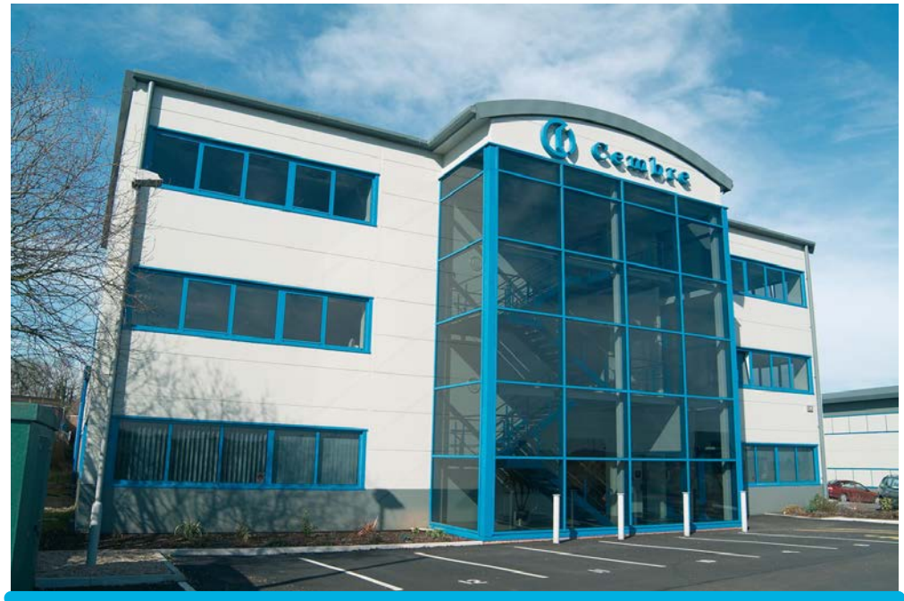
CEMBRE Ltd. – Factory in Curdworth Birmingham (UK)
