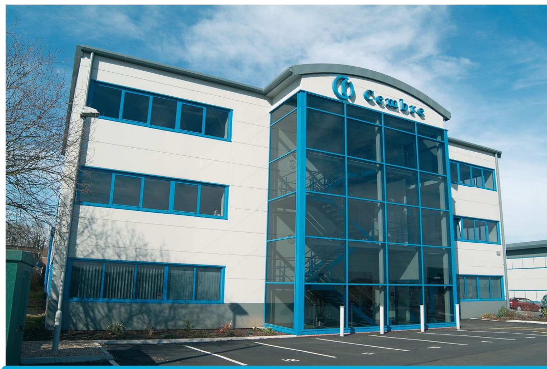
CEMBRE Ltd. – Factory in Curdworth Birmingham (UK)
