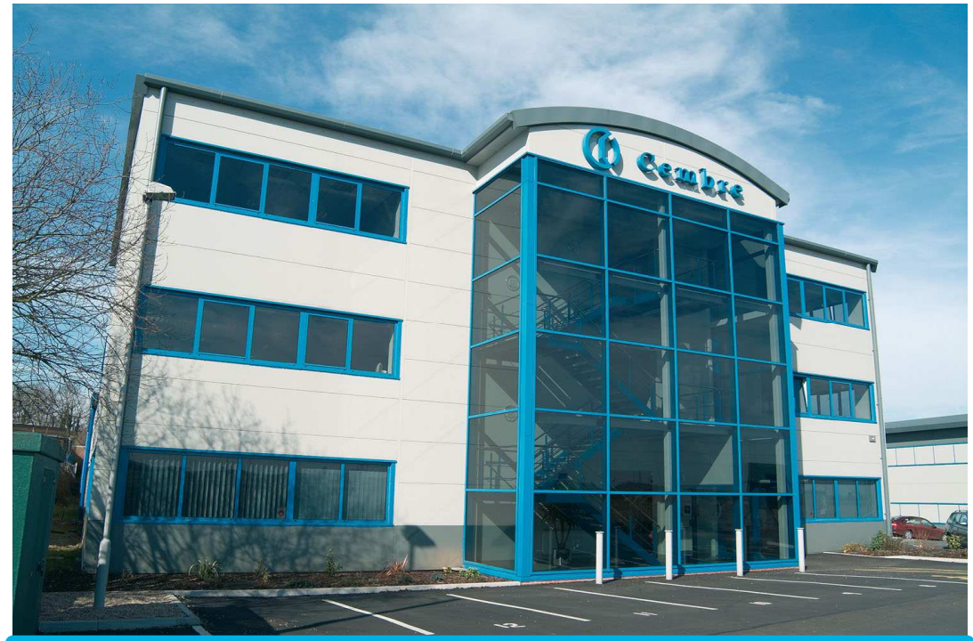
CEMBRE Ltd. – Factory in Curdworth Birmingham (UK)
