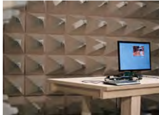
Figure 38: Arezzo plant, interior view of the anechoic chamber
