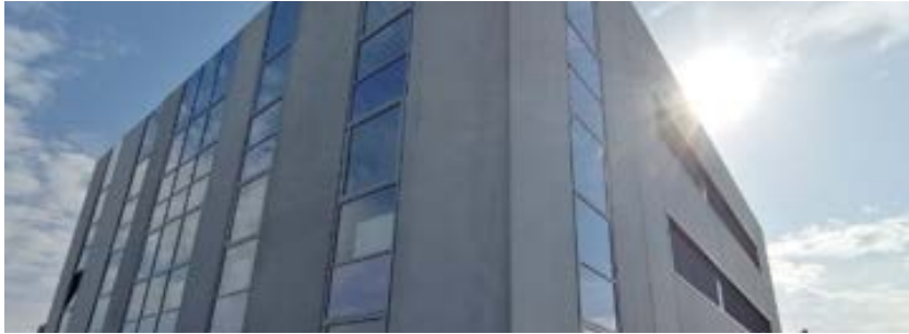
Building of approximately 1,300 square metres on three floors.
