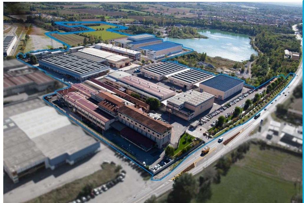
CEMBRE S.p.A. – Headquarter in Brescia (Italy)
