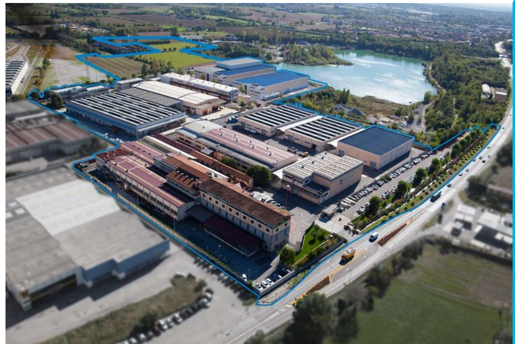
CEMBRE S.p.A. – Headquarter in Brescia (Italy)
