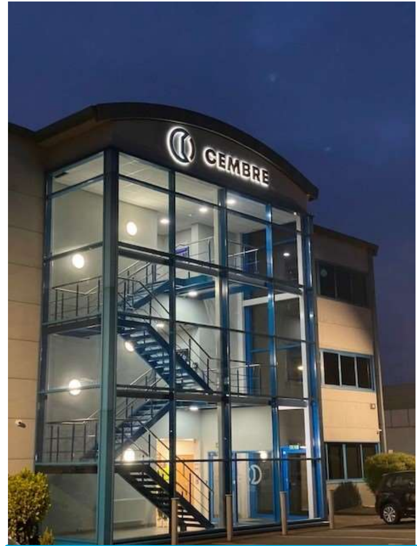
CEMBRE Ltd. – Factory in Curdworth Birmingham (UK)
