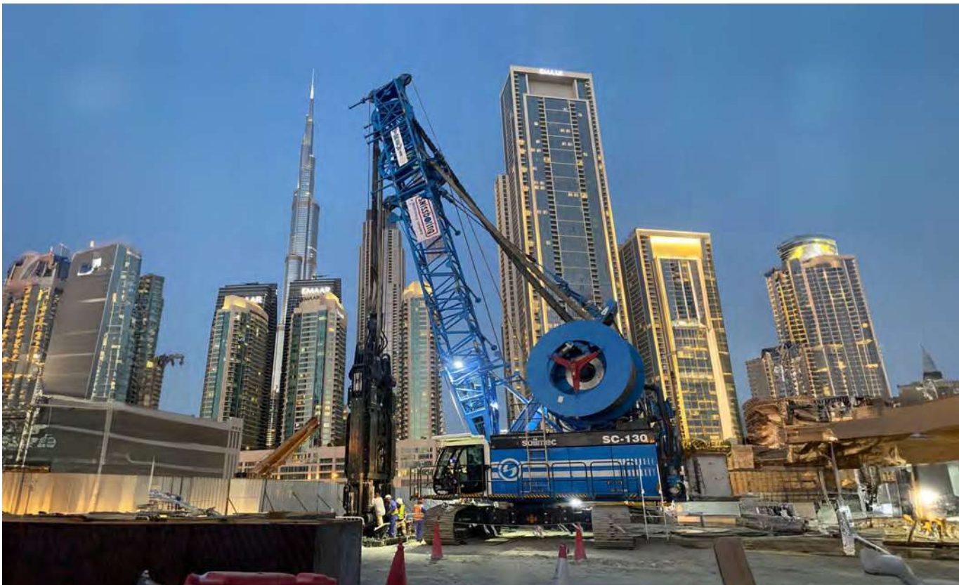
Idrofresa Soilmec, modello "Tiger" SC-130 | Dubai
