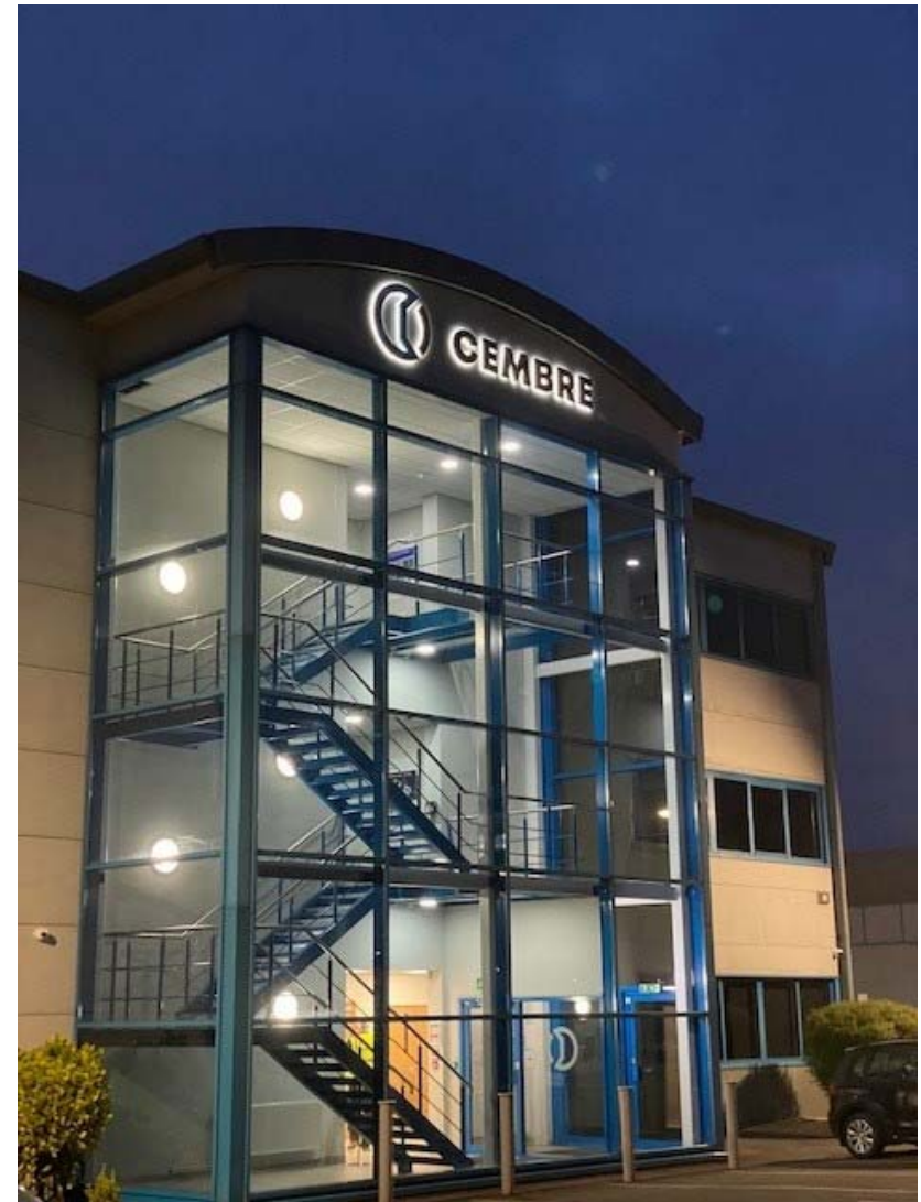
CEMBRE Ltd. – Factory in Curdworth Birmingham (UK)
