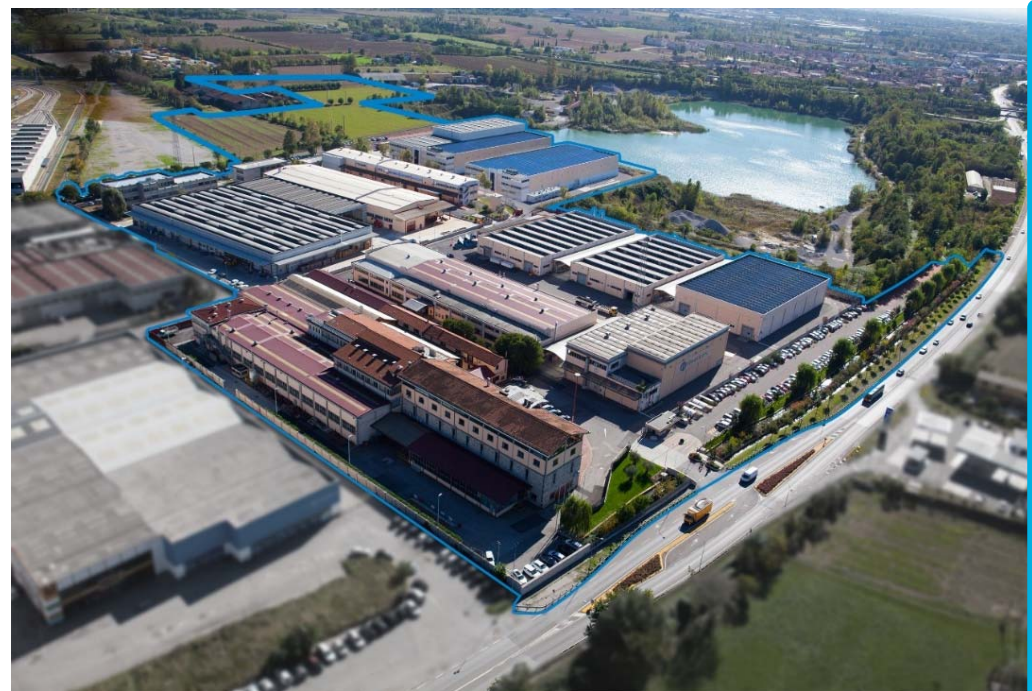
CEMBRE S.p.A. – Headquarter in Brescia (Italy)
