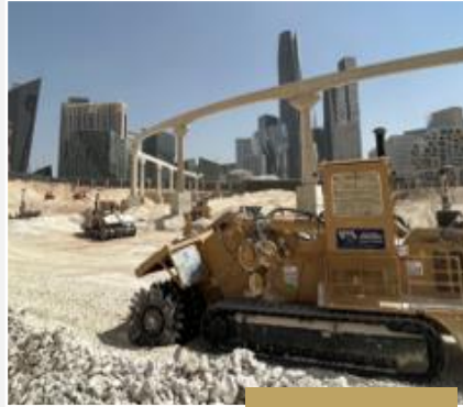
KAFD project – Saudi Arabia
