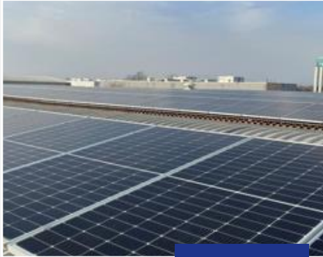
Grassobbio site revamping and extended photovoltaic plant
