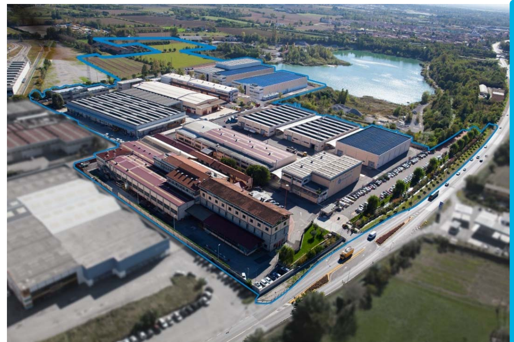
CEMBRE S.p.A. – Headquarter in Brescia (Italy)
