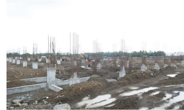
Construction going on in full swing at the 44+ acres new facility
